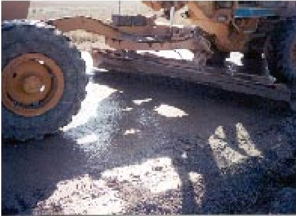
Grader Cutting Road Bed to 4% Crown Section.
