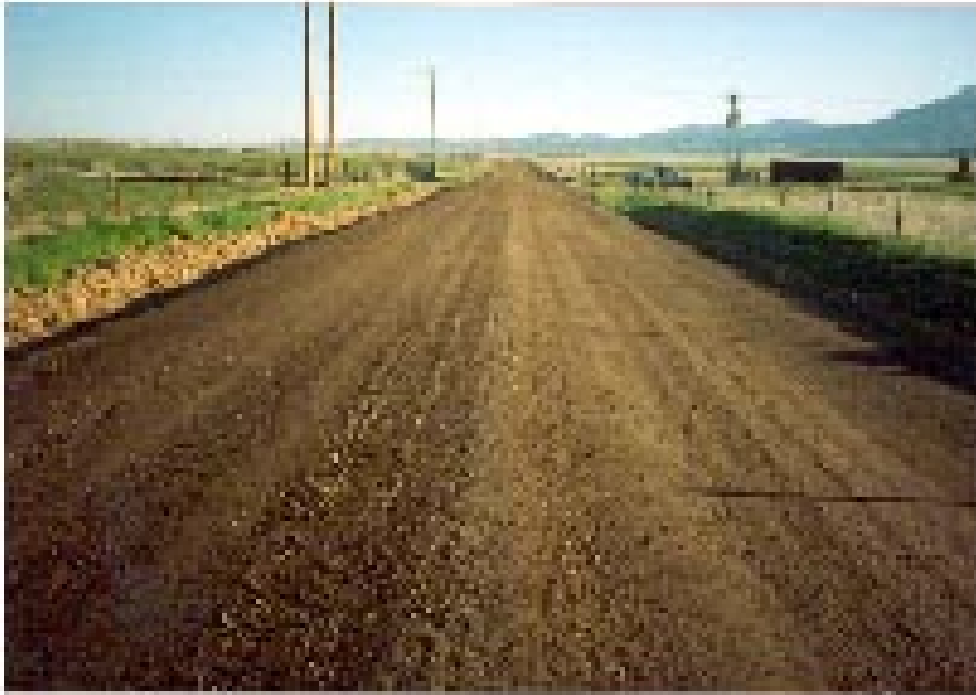
Road Bed Properly Compacted and Prepared for Magnesium Chloride Treatment.
