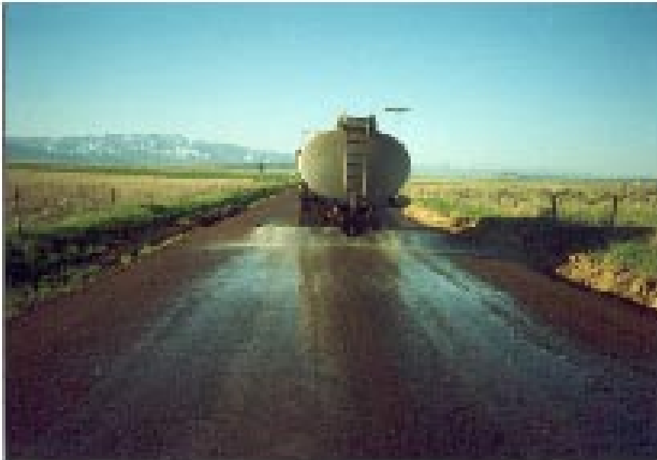
Distributor Truck Applying Magnesium Chloride at 0.5 Gallons per Square Yard.
